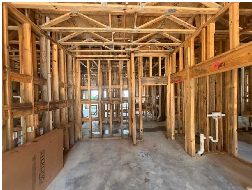
Interior - First Floor: Interior Framing is in place ; Plumbing Rough-ins are in progress.
