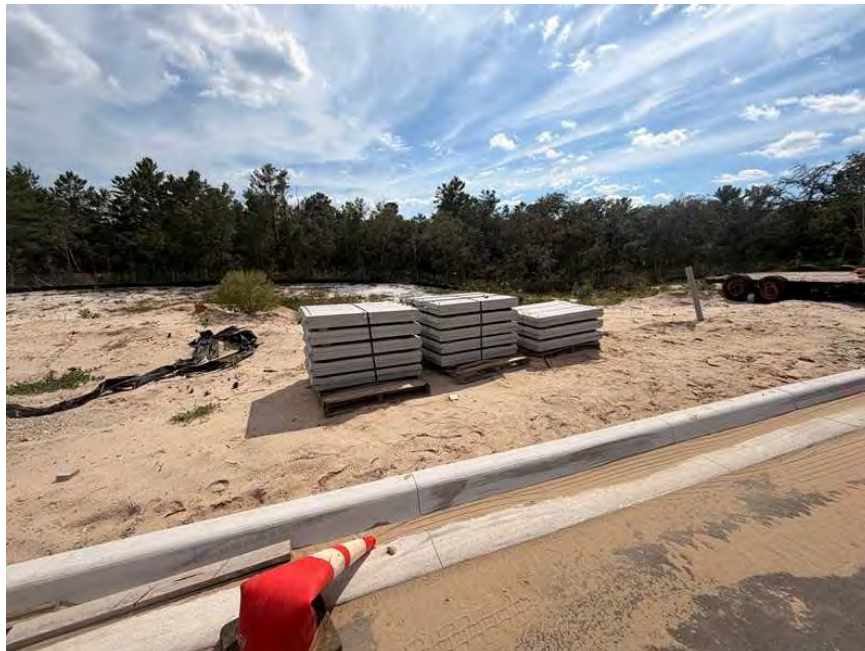
Precast Concrete Treads are stored on site.
