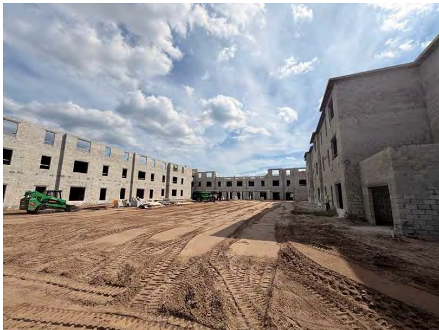
Exterior: CMU Superstructure is in place.
