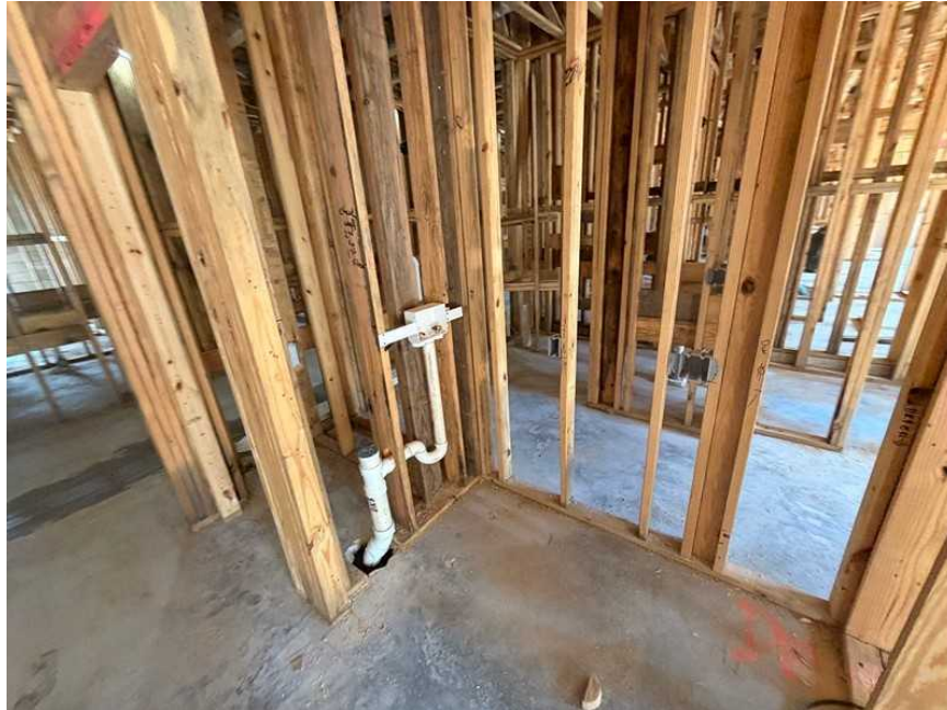
Interior - First Floor: Plumbing Rough-ins are in progress.
