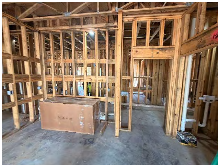
Interior - First Floor: Plumbing Rough-ins are in progress ; Tub is staged.
