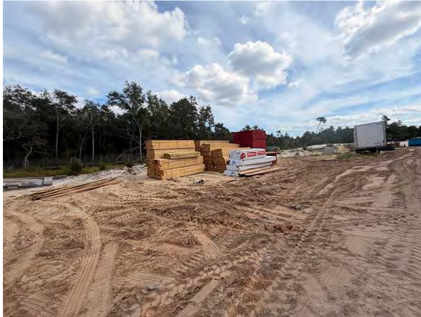
Framing Lumber is stored on site.
