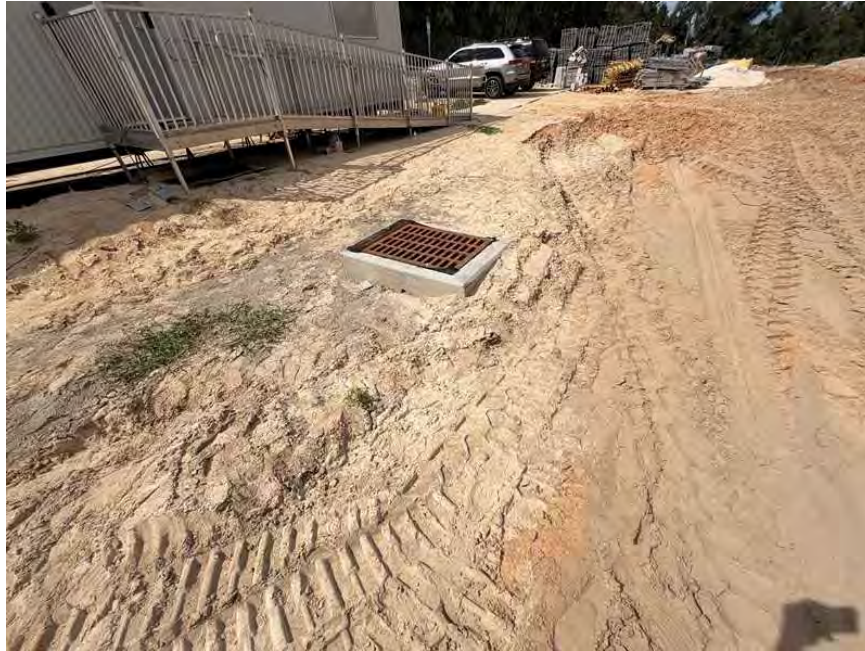
Site: Subsurface Drainage is in place.
