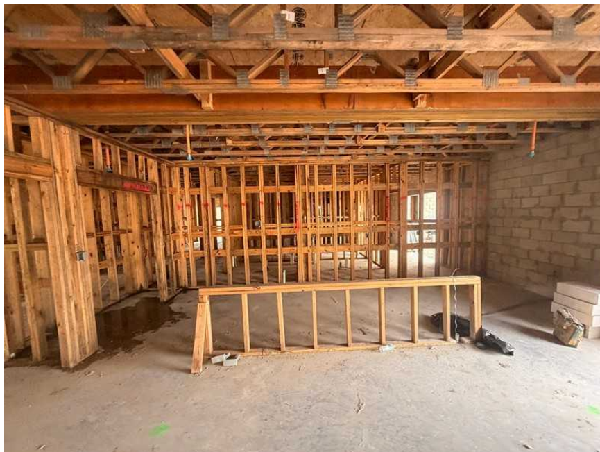
Interior - First Floor: Fire Sprinkler Rough-ins are in progress.
