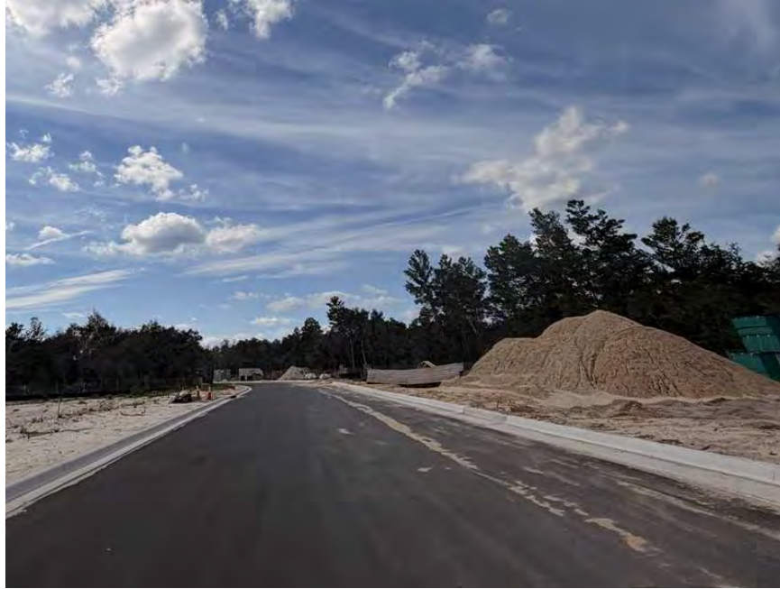
Site: Asphalt Pavement is in place for Roadway Extension.
