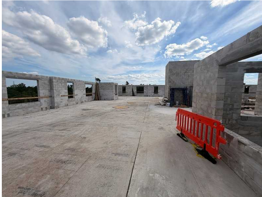
Interior - Third Floor: CMU Superstructure is in place.
