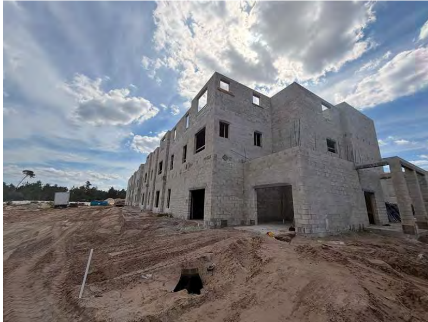
Exterior: CMU Superstructure is in place.
