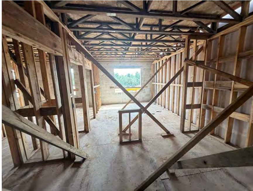
Interior - Second Floor: Interior Framing is in place.
