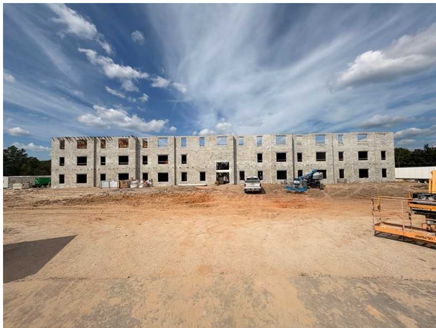
Exterior: CMU Superstructure is in place.
