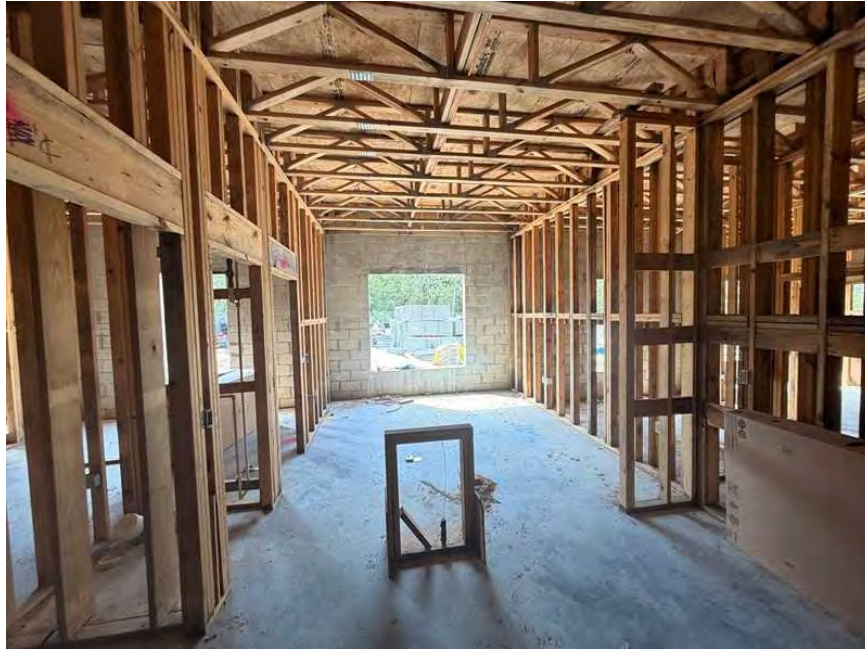
Interior - First Floor: Interior Framing is in place.
